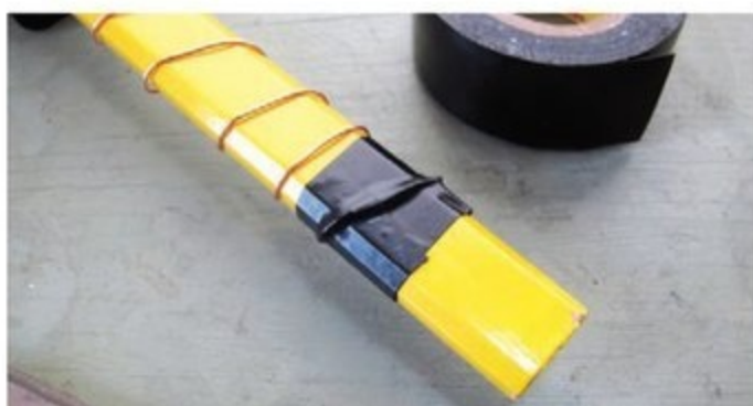
6. Secure the grip lead with electrical tape.
