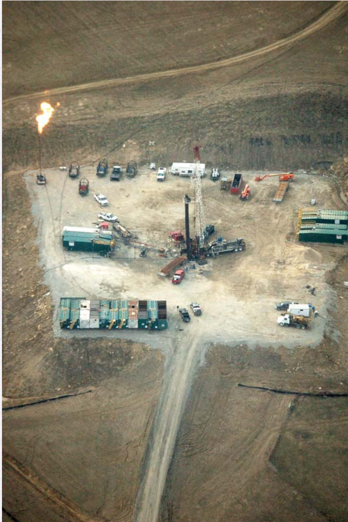
Aerial view of well pad
