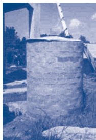
Tank made from stabilised soil blocks in urban Uganda (Picture: T. Thomas)
