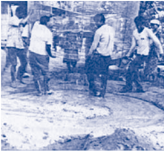
Moving the mould into place
