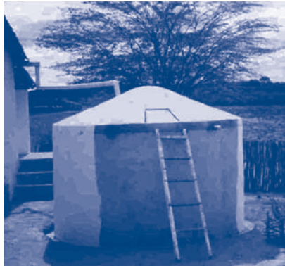
Finished tank being painted
