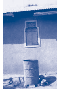
An oil drum tank in rural Uganda (Picture: D. Rees)
