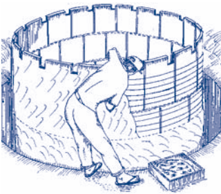
Plastering the outside
