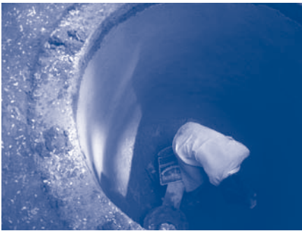
Lining the pit
