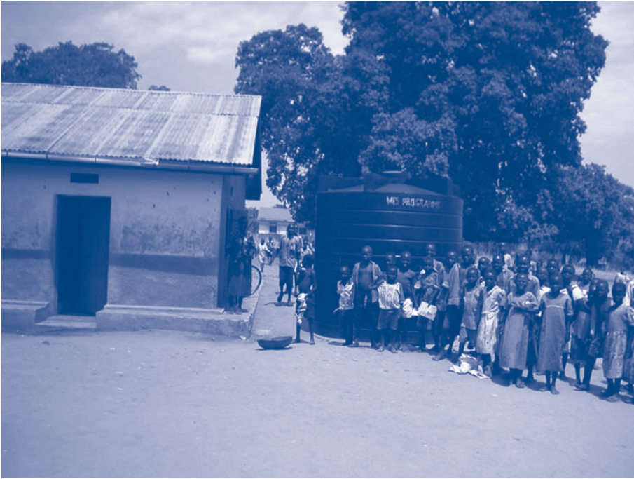
Figure 10.1. Unworkable school system in NW Uganda (Note entrance to the plastic tank is above gutter level)
