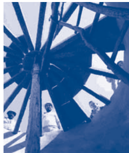
Installing the roof
