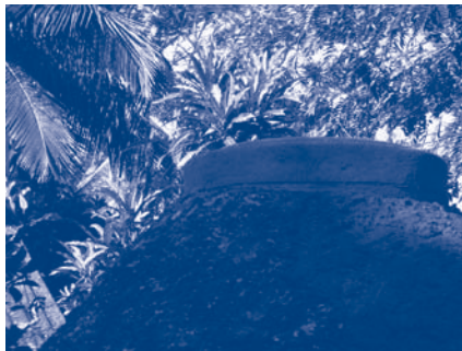
Detail of access to tank
