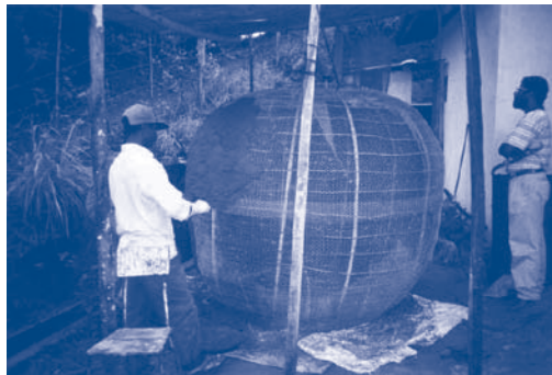
Partially rendered tank
