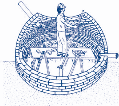
Making the brick dome
