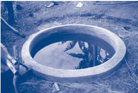
Underground tank with sloped ring beam
