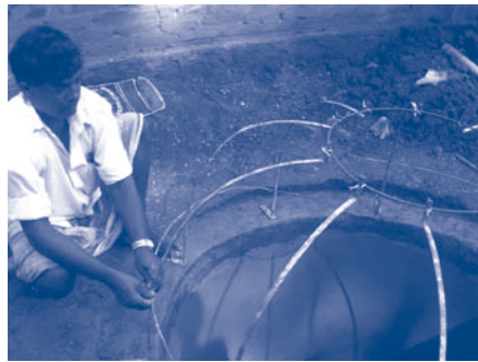
Fixing the frame for the dome
