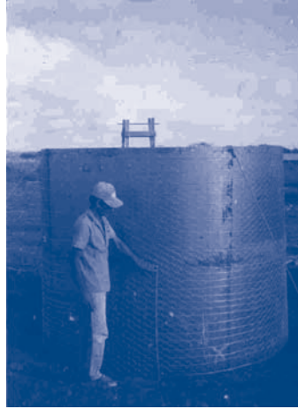
Steel sheet form, wrapped by wire mesh and galvanised wire
