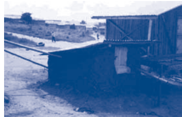
Completed tank (Pictures: D. Rees)
