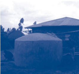
Household ferrocement tank in Ethiopia (Picture: S. Akhter)
