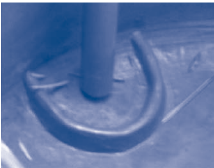
Figure 9.6. Ideal inlet and outlet arrangements (bottom-in top-out) (Diagrams: D.B. Martinson; pictures: D.B. Martinson and V. Whitehead)
