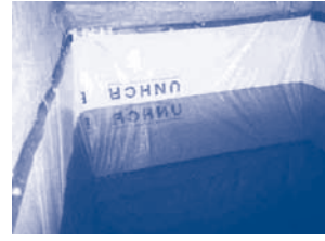
Tarpaulin lined underground tank in rural Uganda (Photo D. Rees)
