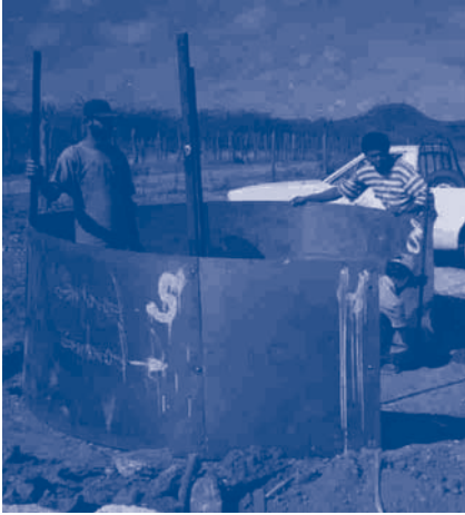
Screwing together the steel sheet form
