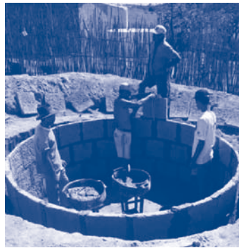
Fixing the plates
