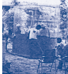
Partially rendered tank
