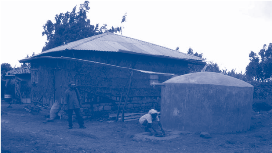
Figure 7.3. Typical rural building in Ethiopia with an unsustainably costly ferrocement tank (Picture: B. Woldemariam)
