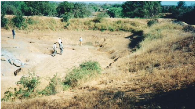
A hillside dam built manually at the foot of a rock outcrop in Kitui, Kenya, some 40 years ago. The dam is still providing clean water for domestic use from a hand-dug well sunk into a seepage line downstream of the dam wall.
