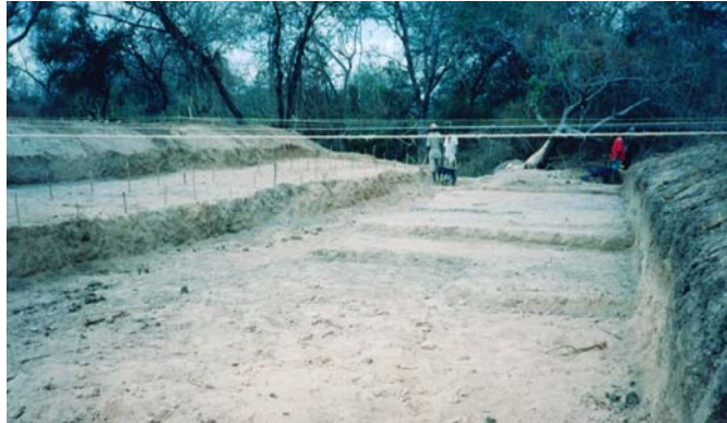
The depth of spillways are measured from nylon strings drawn over the spillways.
