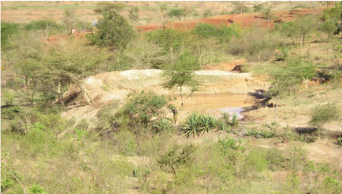
An example of a hillside dam harvesting rainwater run off the Machakos-Kitui road.
