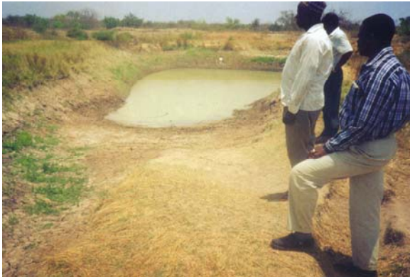
An oval-shaped charco dam on the flat plain west of the Usambara Mountains in Tanzania.
