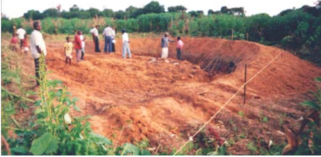
A hillside dam built by a tractor ploughing in circles against the dam wall in Zambia. It took the farmer two weeks to complete the construction works.
