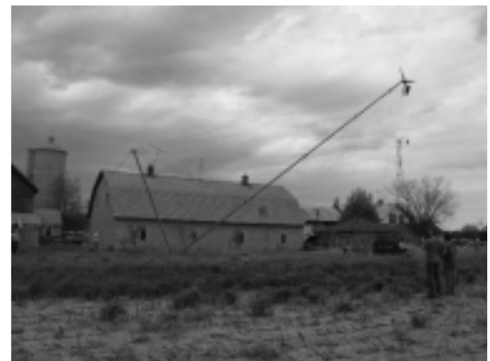
Figure 27 - A tilt-up tower halfway raised.
