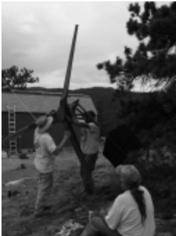
Figure 53 - Balancing the blades while on the tower stub.
