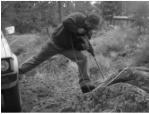
Figure 34 - Drilling out a rock formation for a guy wire anchor.
