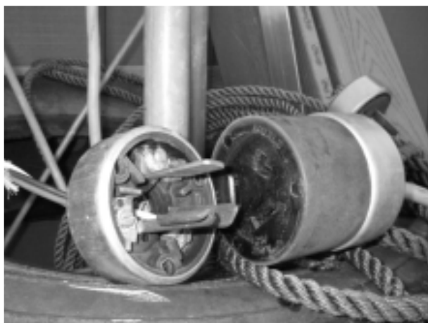
Figure 20 - Locking plug and socket at the tower base.
