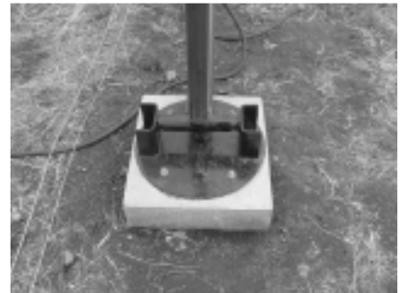
Figure 32 - A simple tower base and hinge.
