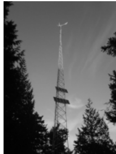
Figure 23 - Freestanding lattice tower with both wind turbine and solar panels mounted on it.
