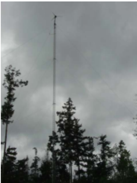
Figure 24 - A 140 foot guyed lattice tower with 12 foot diameter wind turbine flying.
