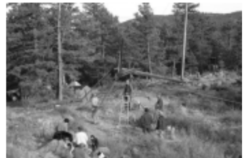
Figure 55 - Preparing to raise the wind turbine.
