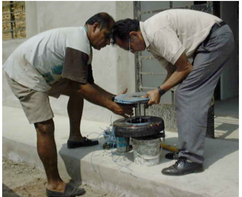
On site assembly in Peru
